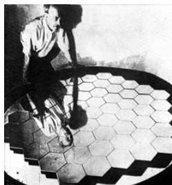
Guido Horn d'Arturo at Bologna Observatory Built between 1935-52 61 segments to form 1.8m diameter mirror
